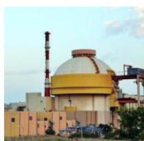
The reported data leak comes amid construction of four VVER reactors at the plant. FILE PHOTO
