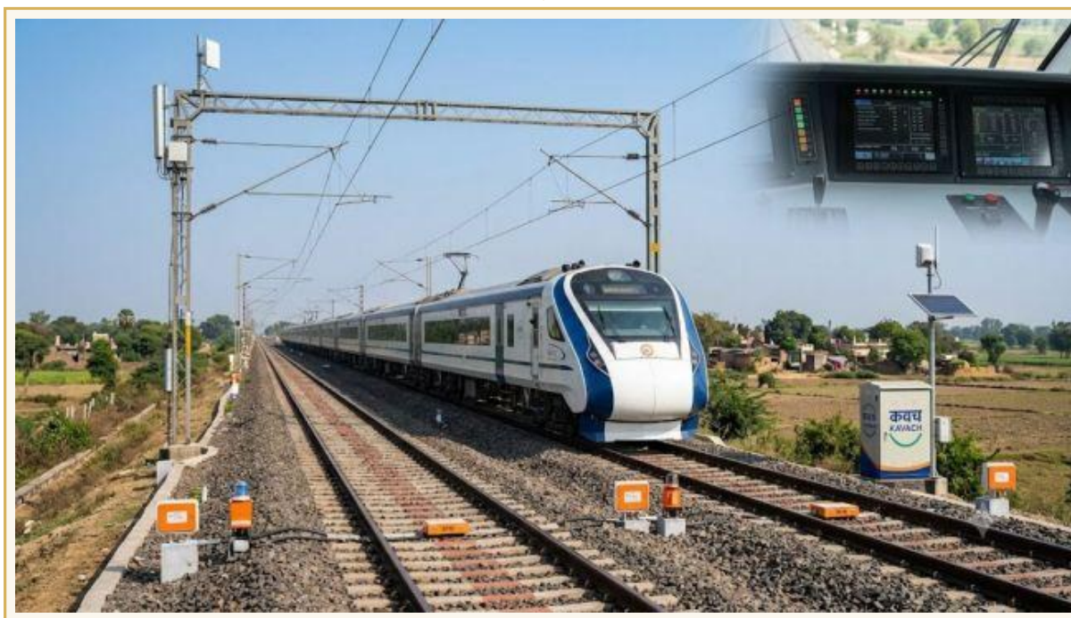
Kavach — RFID tags on track, lineside tower and loco cab display
